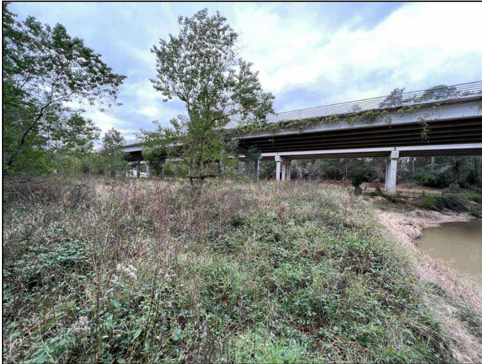
Photograph 13 –View of Gosling Road overpass near the northwestern corner of the Subject Property, facing southwest.
